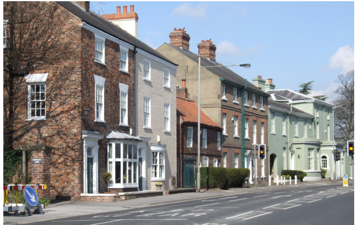
Traditional buildings in Main Street, near Heslington Lane Junction
