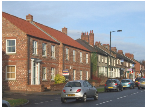
St. Oswald’s Court housing development
