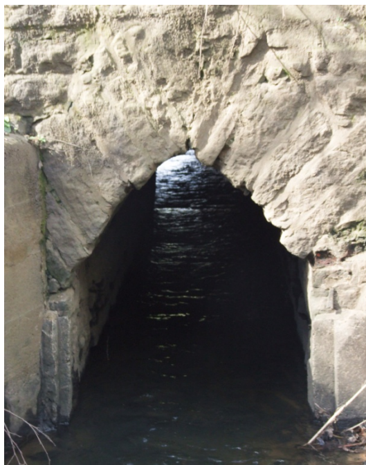
Original pointed arch stone bridge
